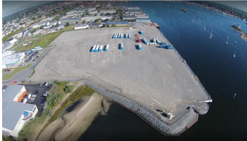
Figure 9-20 New Bedford Marine Commerce Terminal
