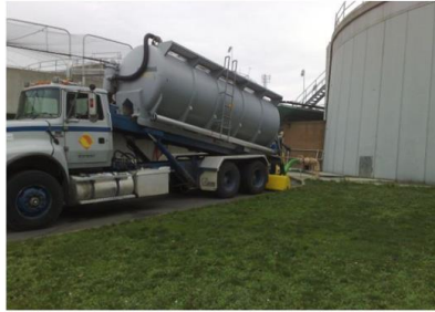
Trucked waste offloading at Iona Island WWTP
