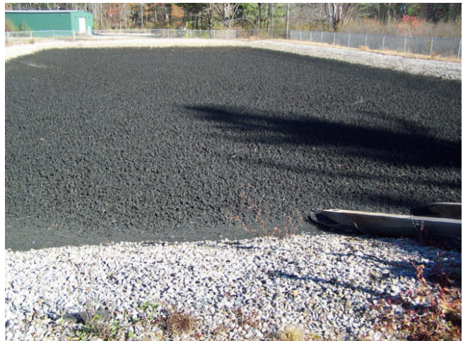
A wastewater solids (sludge) solids dewatering lagoon
