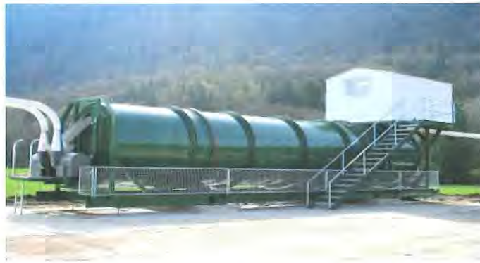
Figure 10: Ecodrum with air handling system
